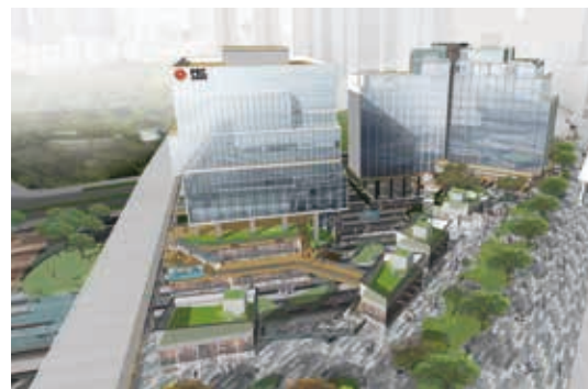
The overview of Dorsett Kai Tak, Hong Kong
