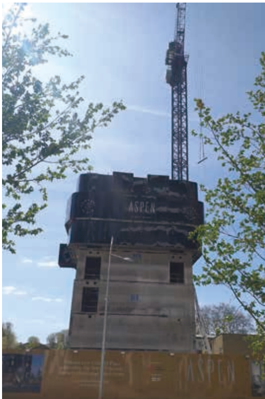
The construction site, Aspen at Consort Place, London
