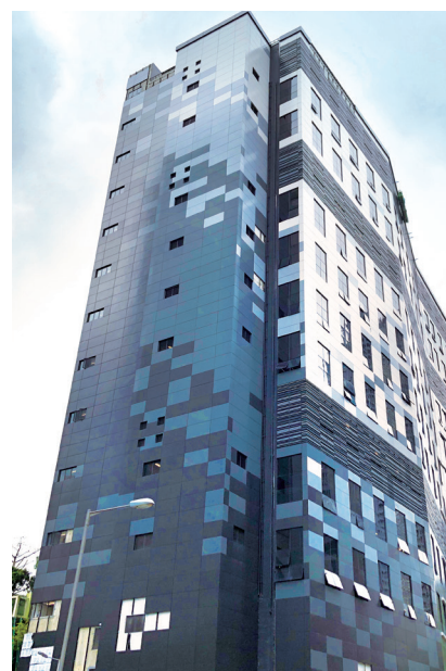
Data Centre, 11 Kin Chuen Street
