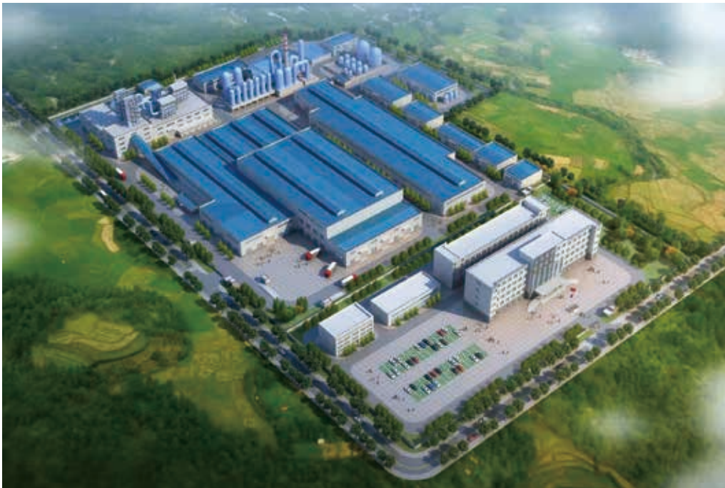
Tianneng Circular Economy Industrial Park in Anhui Province
