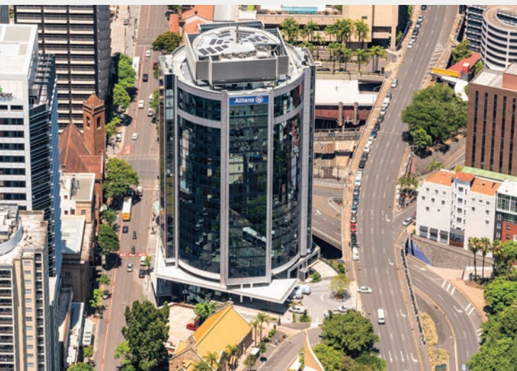
Australia Office Building 澳洲寫字樓, Brisbane 布里斯班
