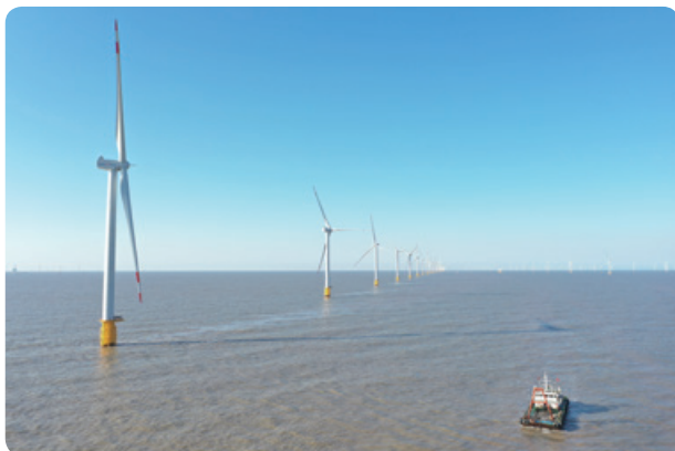
Rudong H8# offshore wind power project (300 MW) in Jiangsu Province 江蘇省如東H8#海上風電項目(300兆瓦)
