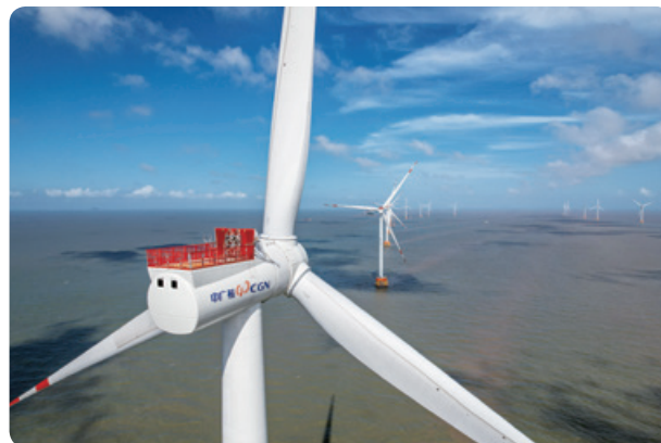
Shengsi 5# and 6# offshore wind power project (281.25 MW) in Zhejiang Province 浙江省嵎泗5#、6#海上風電項目(281.25兆瓦)
