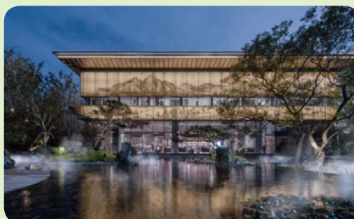
Shanghai Jinyuewan Project
