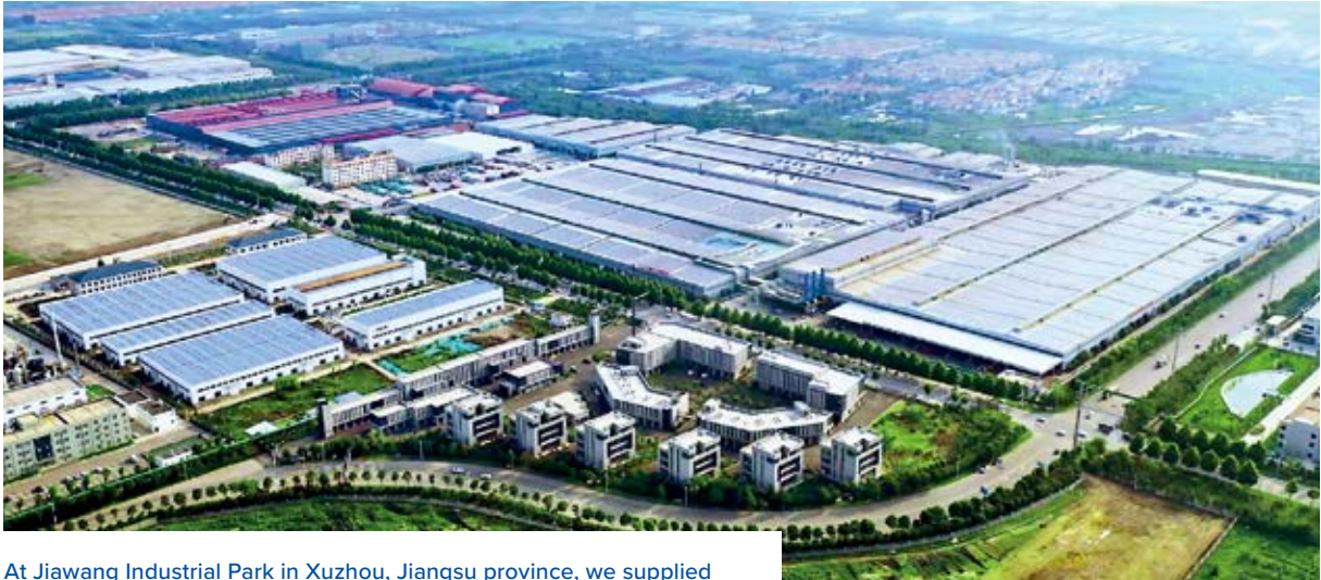
At Jiawang Industrial Park in Xuzhou, Jiangsu province, we supplied steam heat to local residents and businesses as a replacement for coal.
