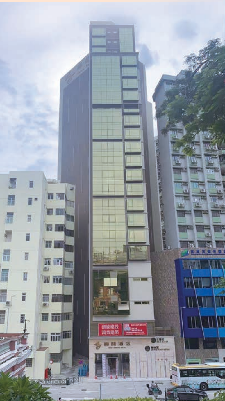
Construction works for a hotel situated on a parcel of land at No.5-11, Travessa do Comandante Mata e Oliveira, Macau
