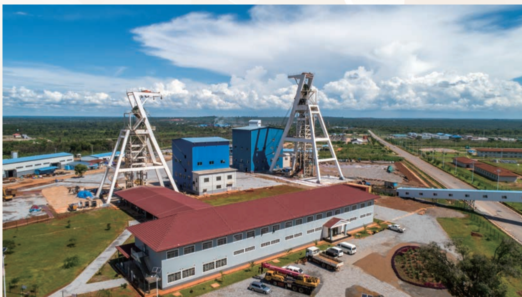
Main and auxiliary shafts of NCA Southeast Mine
