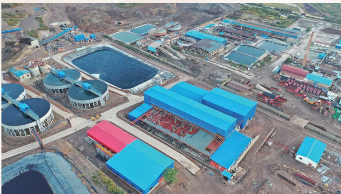
Huachin Leach Plant Area
