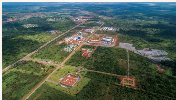
General View of NFCA Southeast Mine
