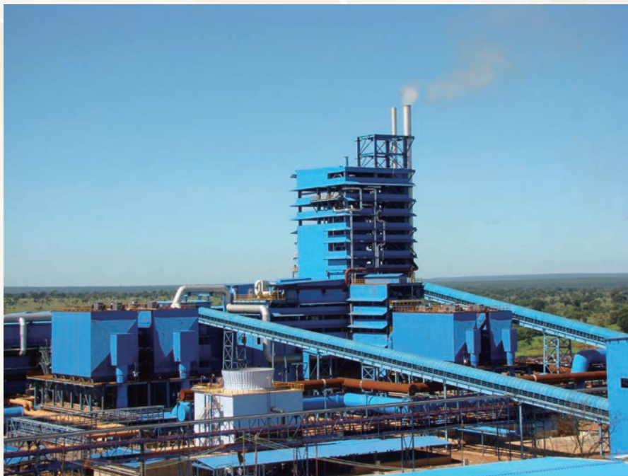
Full view of Isasmelt furnace at CCS
