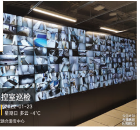
Grandstand Fire Services Central Control Room
