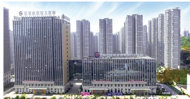
Hospital property services for Guiyang Yuecheng Women's and Children's Hospital
