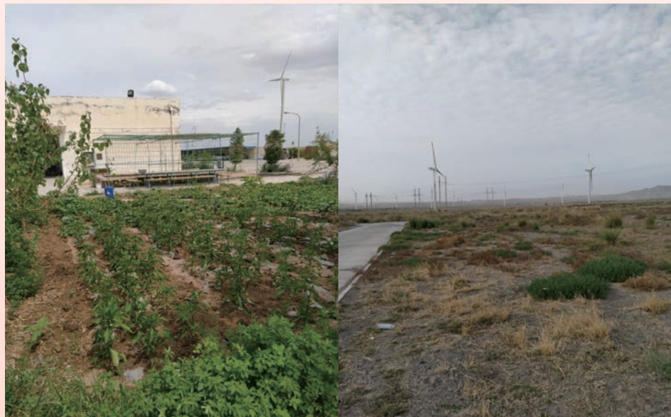
Greening inside and outside the wind farm of Datang Gansu Renewable Power Company Limited
