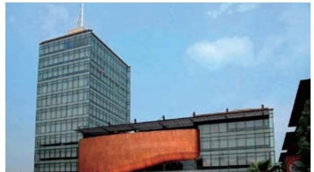
Data Center of Agricultural Bank of China
