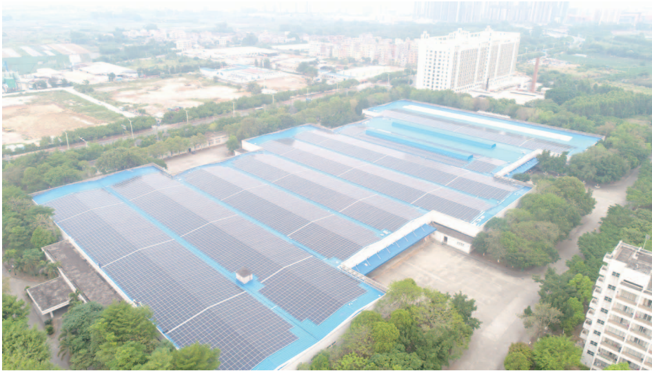
Phase I of the photovoltaic power generation facilities of the Huizhou Factories
