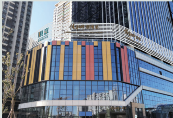
New commercial building at Kunming City, Yunnan Province, with Carrianna Chao Zhou cuisine and "Shunyi" Shunde cuisine restaurant and mooncake exhibition centre 於雲南省昆明市之新置商業大廈·內設佳寧娜潮州菜和「順意」順德菜館及月餅展銷中心
