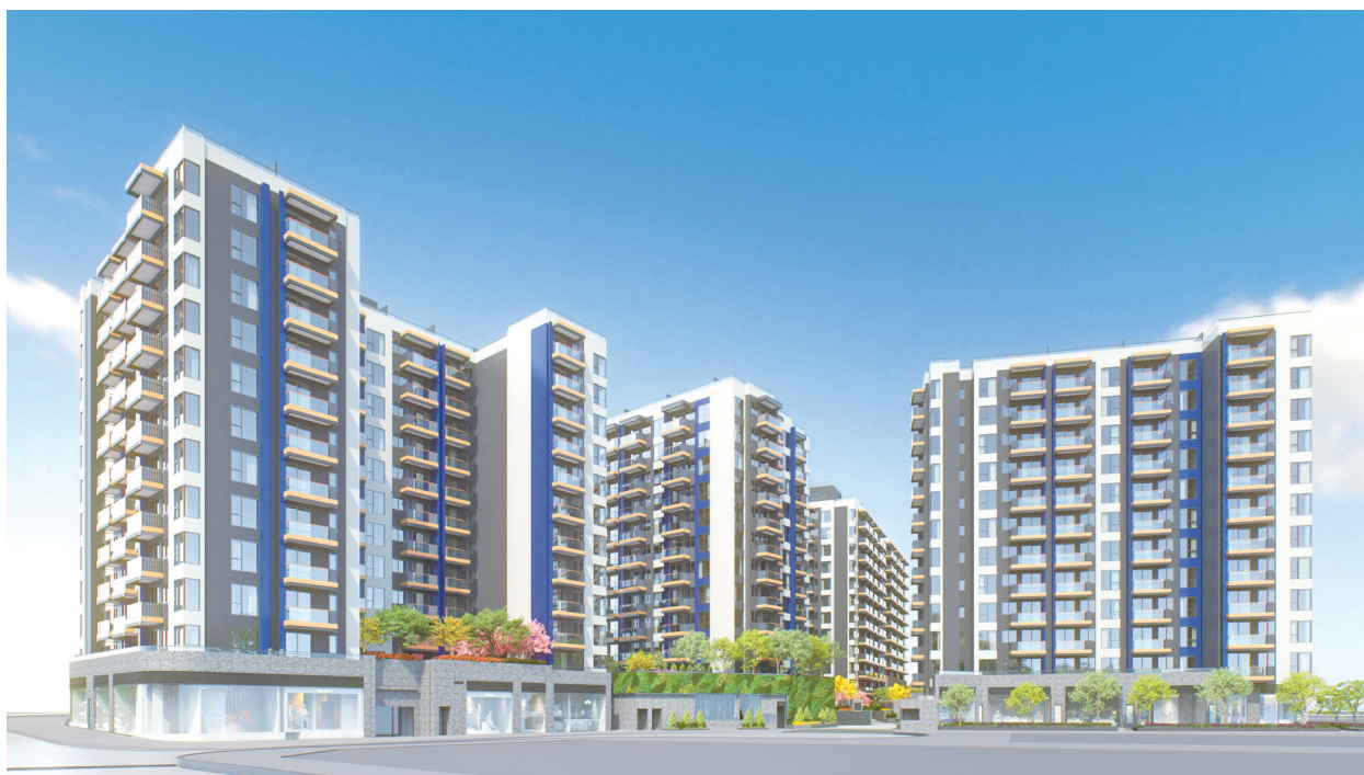
Residential development at Hung Shui Kiu
