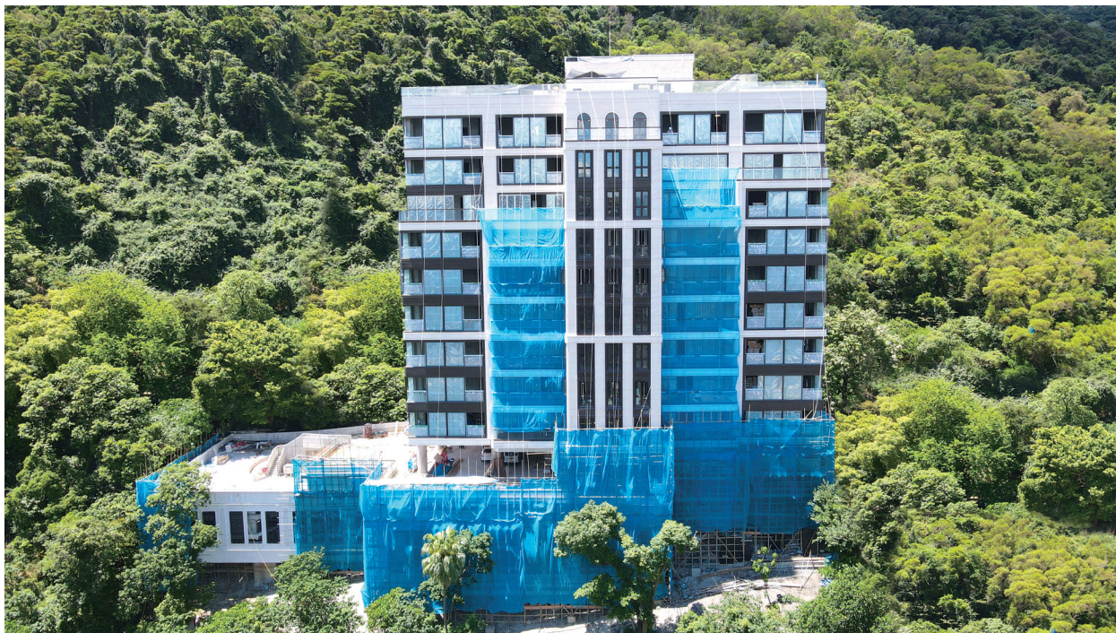
Residential development at Po Shan Road
