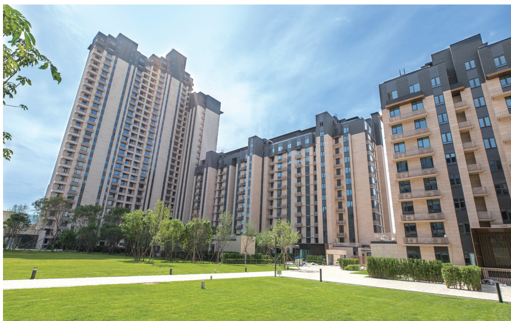
Development project "Capital Cove" in Tongzhou, Beijing
