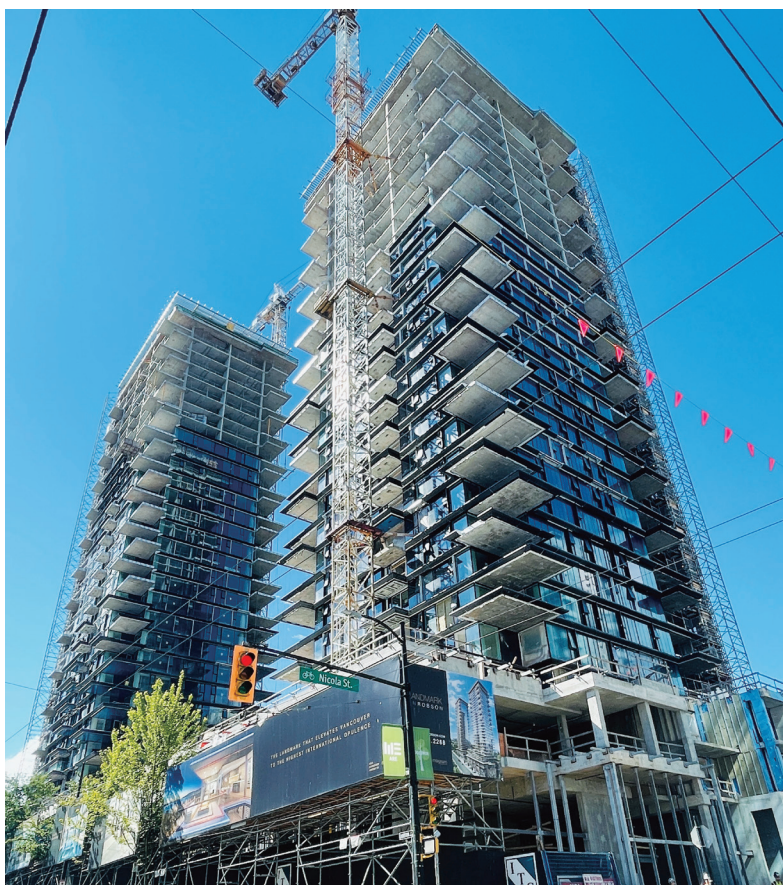
"Landmark on Robson": topped out in May 2022
