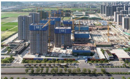
Construction Site of Hangzhou North Star • Chunlan Mansion
