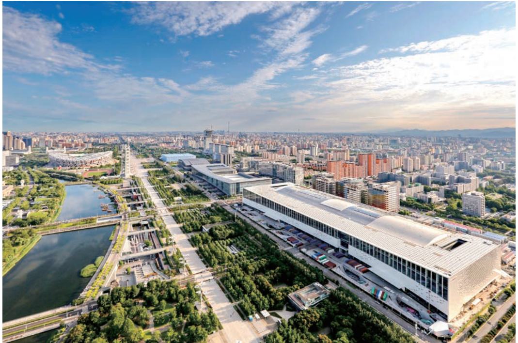
Main Media Center for the Winter Olympics
