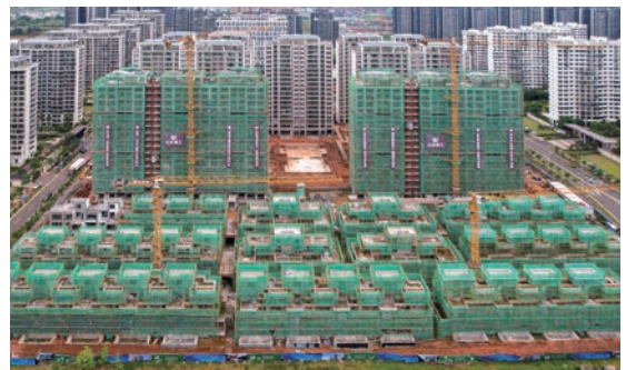
Construction Site of North Star Mansion in Haikou
