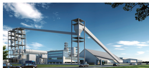
Suining Anju Lithium Carbonate Plant (under construction)
