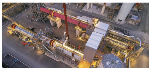
Western Australia Kwinana Lithium Hydroxide Plant
