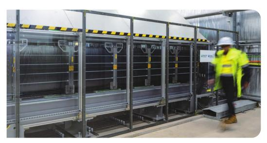
MAGN's zero-emissions 1.25-MW electrolysis plant in South Australia creates green hydrogen and enables completely zero-carbon heating.
