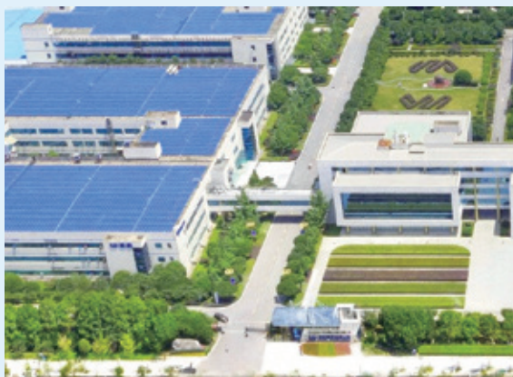
Part of factories in production base of Wasion Group Limited
