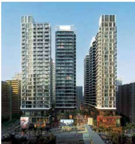
Various projects spanning Gillies Avenue South, Baker Street and Whampoa Street, Hung Hom, Hong Kong (artist's impression)
