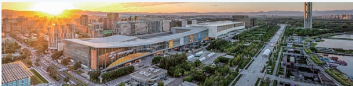
Exterior of Phase I and Phase II of the National Convention Center during CIFTIS 2022
