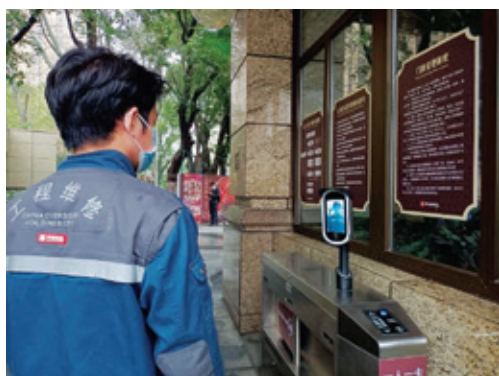
Intelligent access control to save manpower
