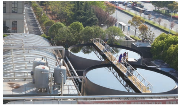
Second Sedimentation Tank for Reclaimed Water Reuse of Yadong (Changzhou)
