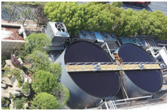
Second Sedimentation Tank for Reclaimed Water Reuse of Yadong (Changzhou)
