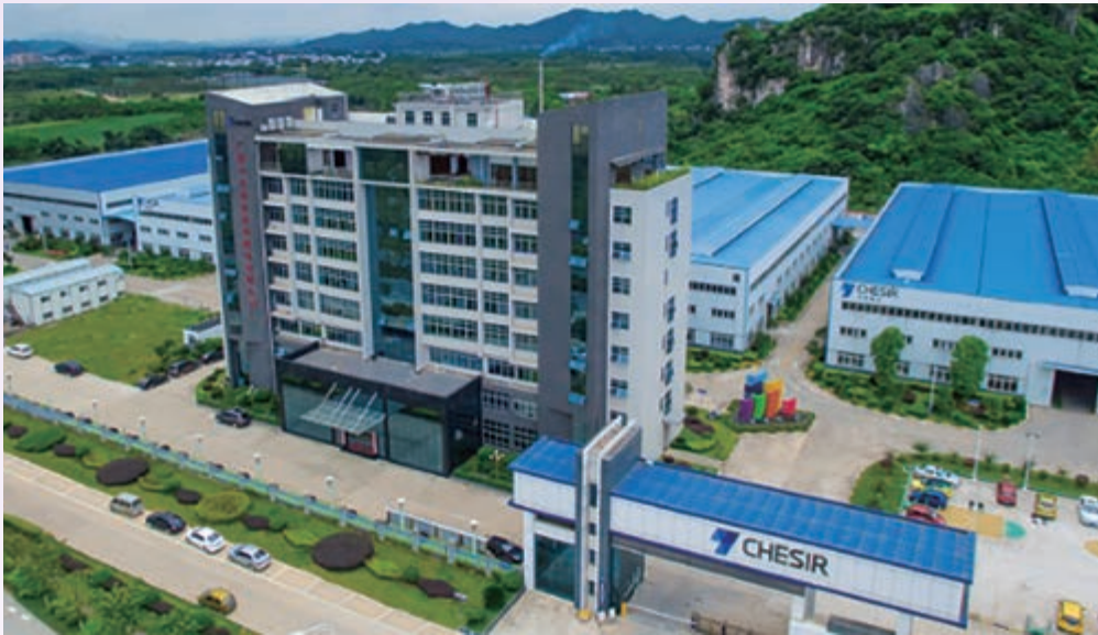
The rooftop distributed photovoltaic project site
