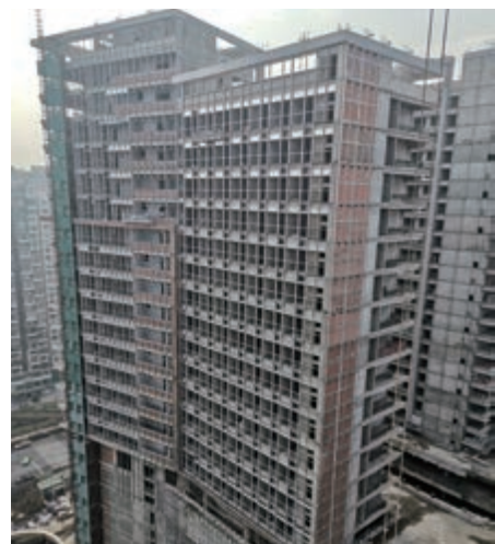
Superstructure works for the commercial/office towers of Regal Cosmopolitan City in progress
