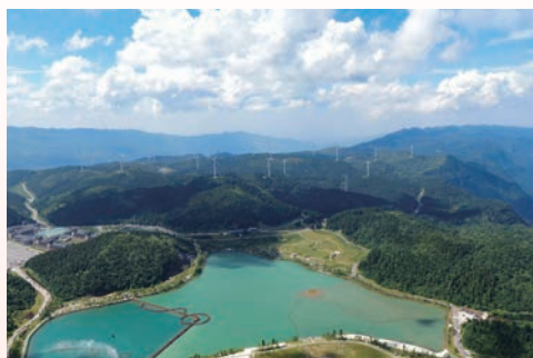
Fengdu Sanba Wind Farm
