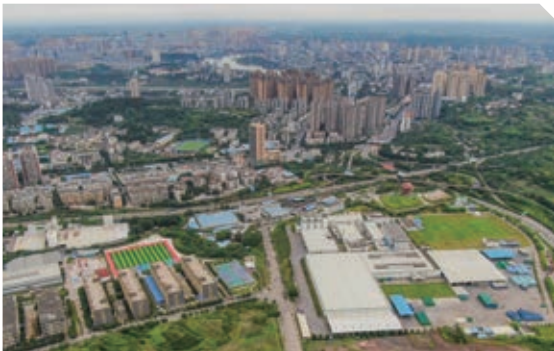
Neijiang Economic Development Zone sanitation project
