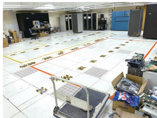
Space is freed up after dismantling network equipment.
