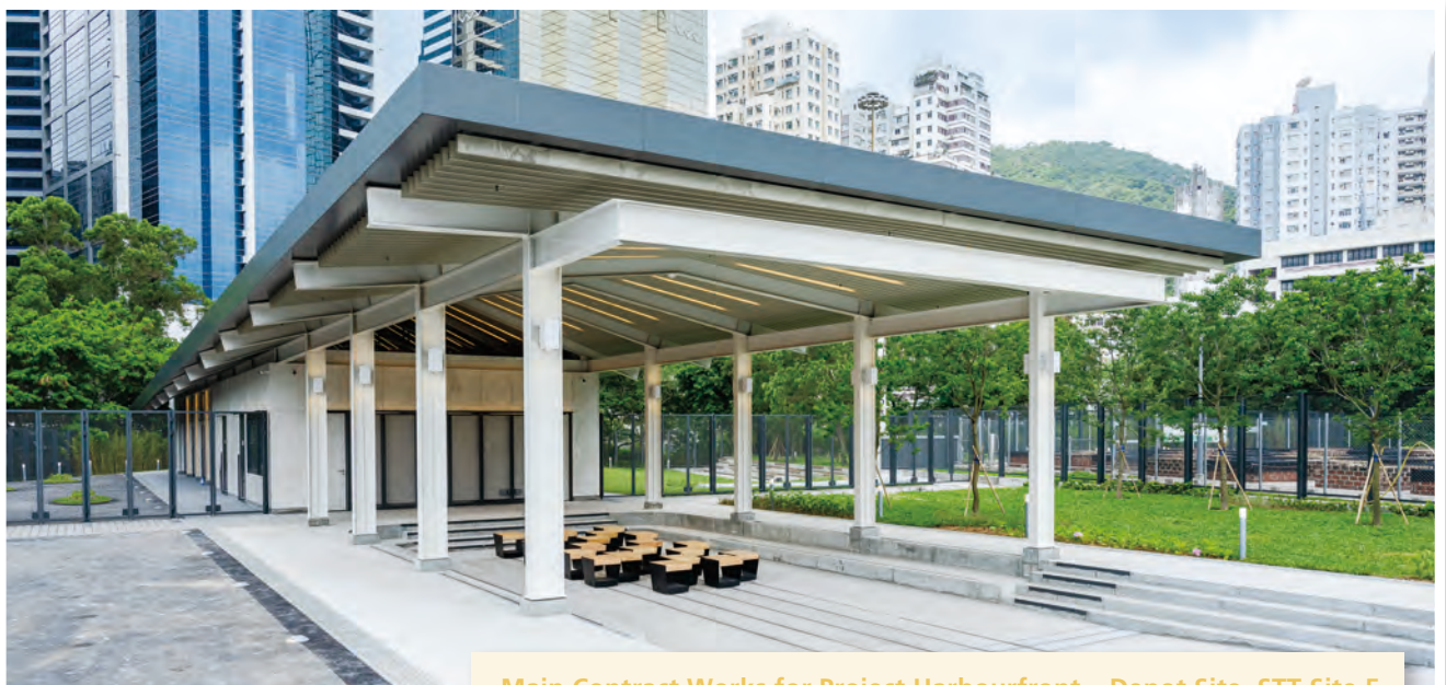
Main Contract Works for Project Harbourfront – Depot Site, STT Site 5 Development at Quarry Bay, Hong Kong 海濱工程項目主合約：香港鰂魚涌第五號短期土地發展臨時用地
