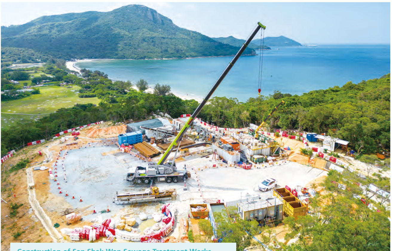
Construction of San Shek Wan Sewage Treatment Works, Associated Submarine Outfall and Pui O Sewerage Works 礮石灣污水處理廠、相關海底排放管及貝澳污水收集系統建造工程
