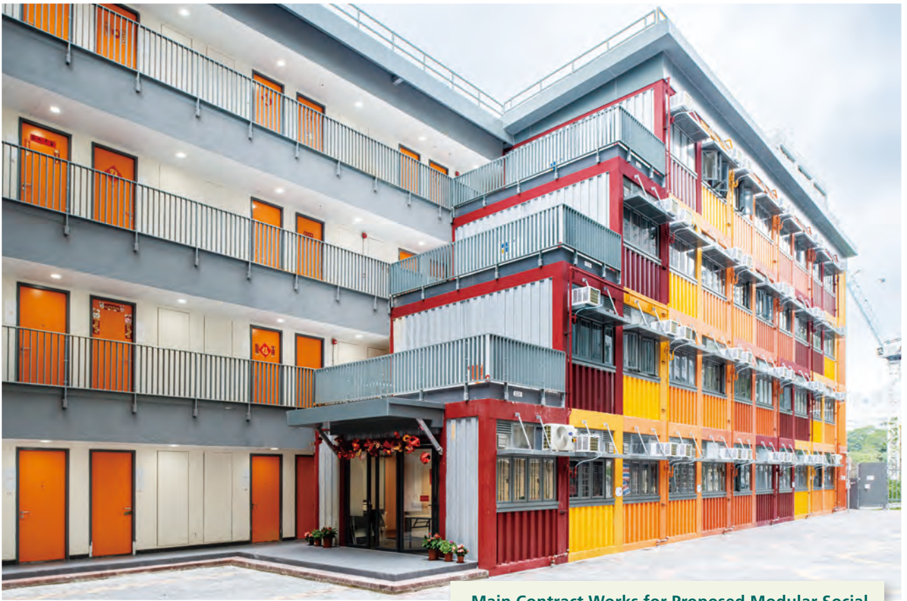
Main Contract Works for Proposed Modular Social Housing at 5-7 Yip Shing Street, Kwai Chung 葵涌業成街5-7號組合社會房屋項目
