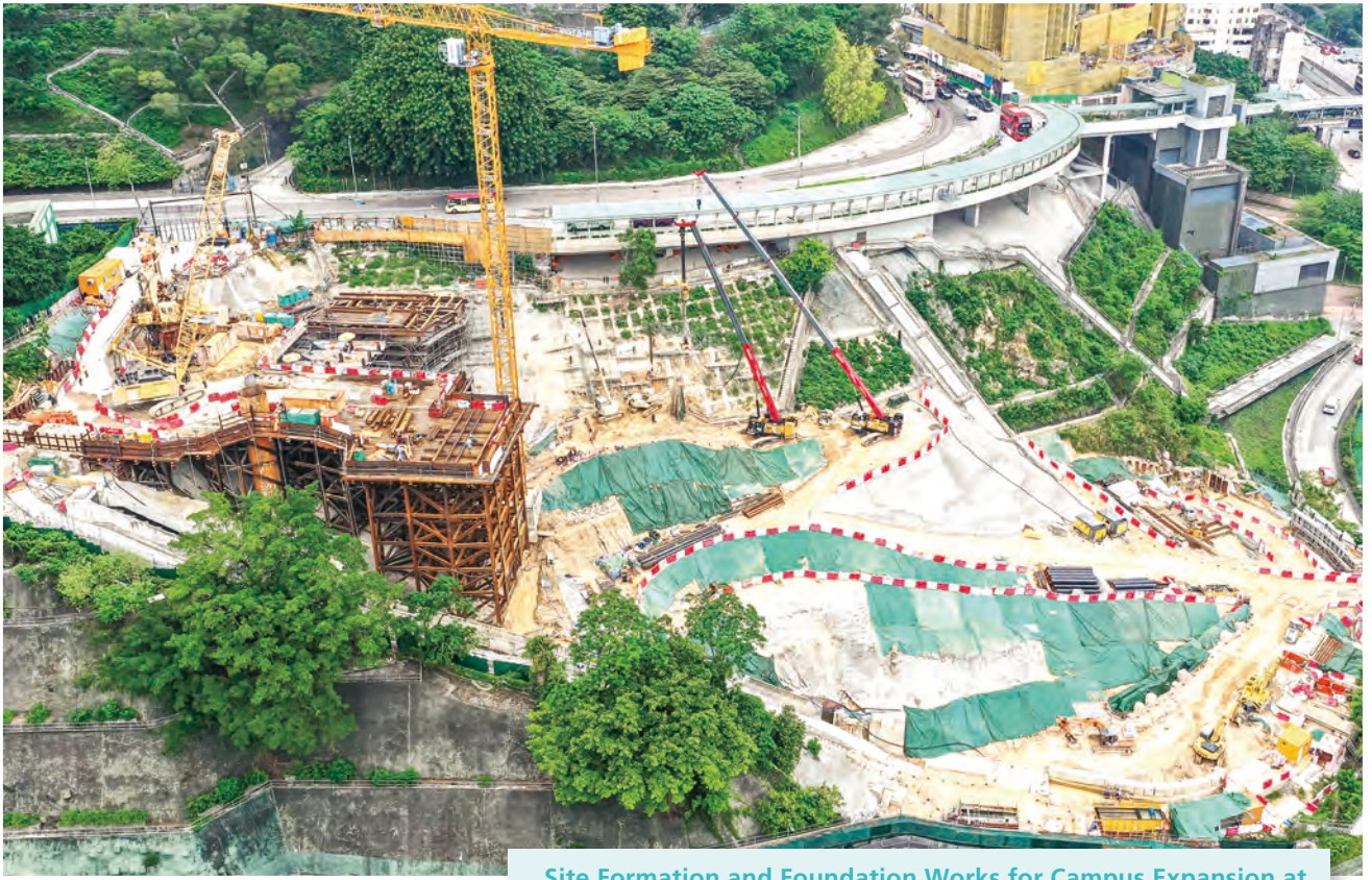
Site Formation and Foundation Works for Campus Expansion at Ho Man Tin Slope for the Hong Kong Polytechnic University 香港理工大學何文田斜坡校園擴建的地盤平整及地基工程
