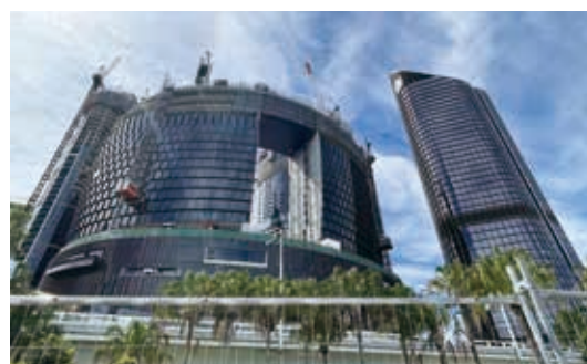
Construction at Queen's Wharf Brisbane
