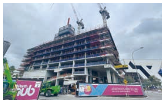
Construction at Perth City Link
