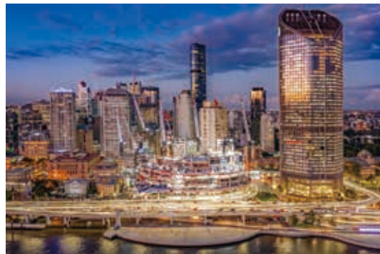
Construction at Queen's Wharf Brisbane
