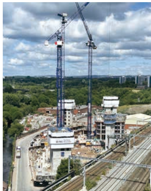
Construction at Victoria Riverside, Manchester
