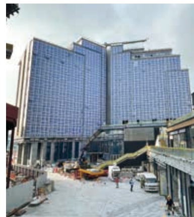
Construction at Dorsett Kai Tak, Hong Kong
