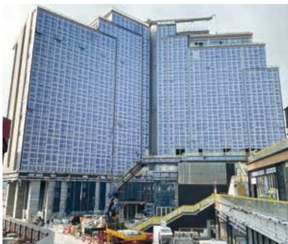
Construction at Dorsett Kai Tak, Hong Kong
