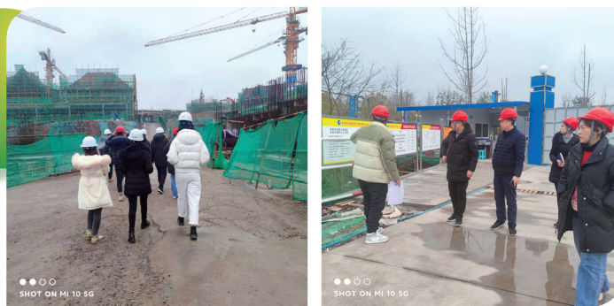
Safety inspection of the Property development business 物業發展業務安全檢查
