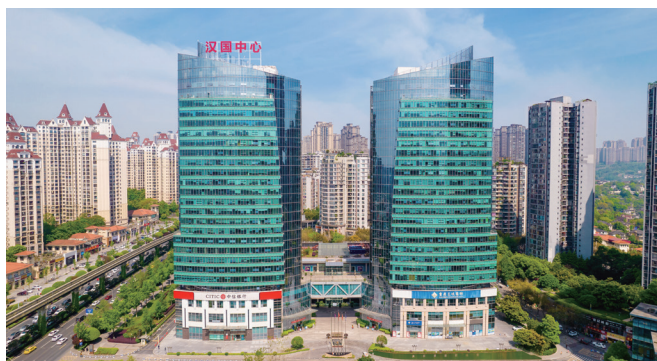
Chongqing Hon Kwok Centre
