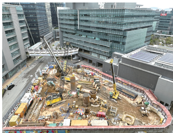
Foundation piling works at Hong Kong Science Park
