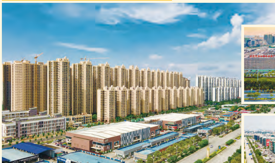
▲ Commercial Complex 1668 Square and Residential Ancillary (Jiangnanhuafu) in CSC Nanning ▲ 南寧華南城的商業綜合體1668廣場及住宅配套(江南華府)
