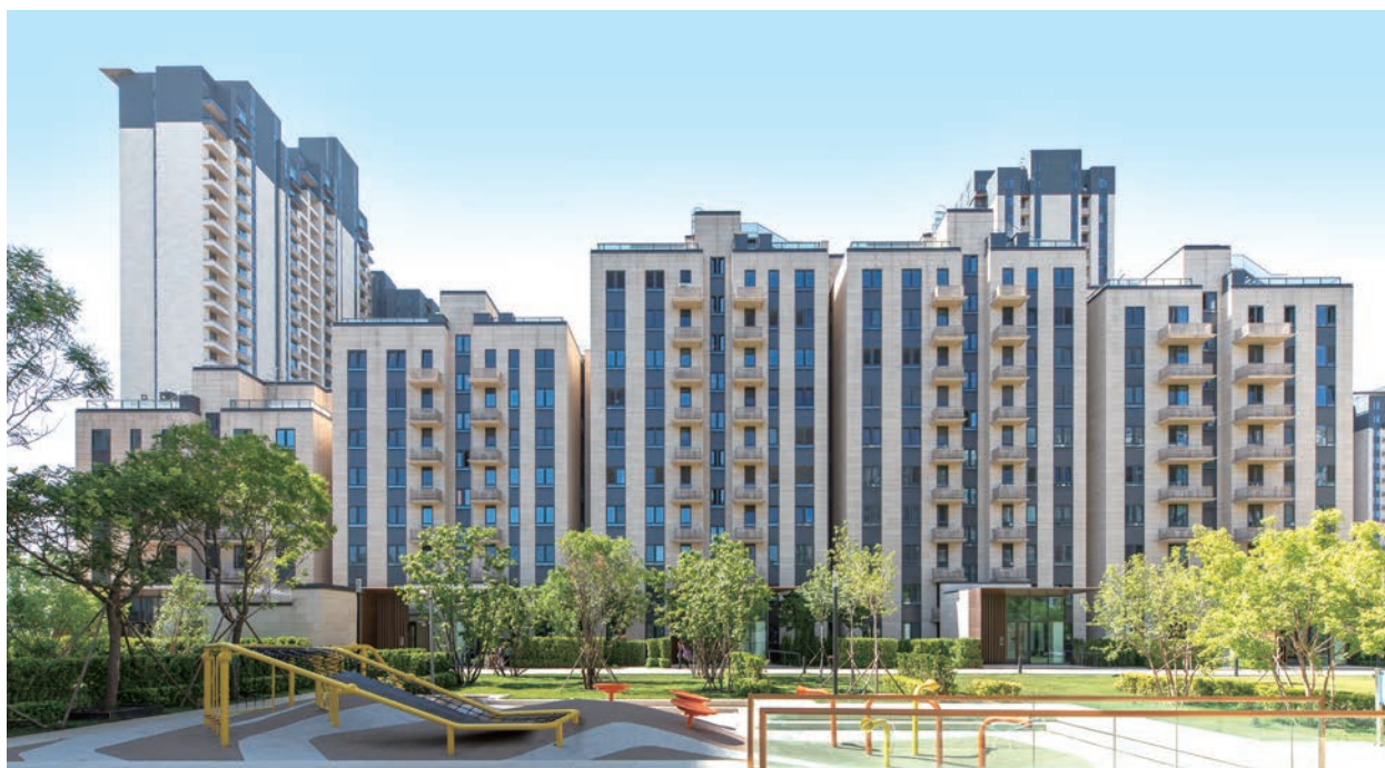
Development project "Capital Cove" in Tongzhou, Beijing
