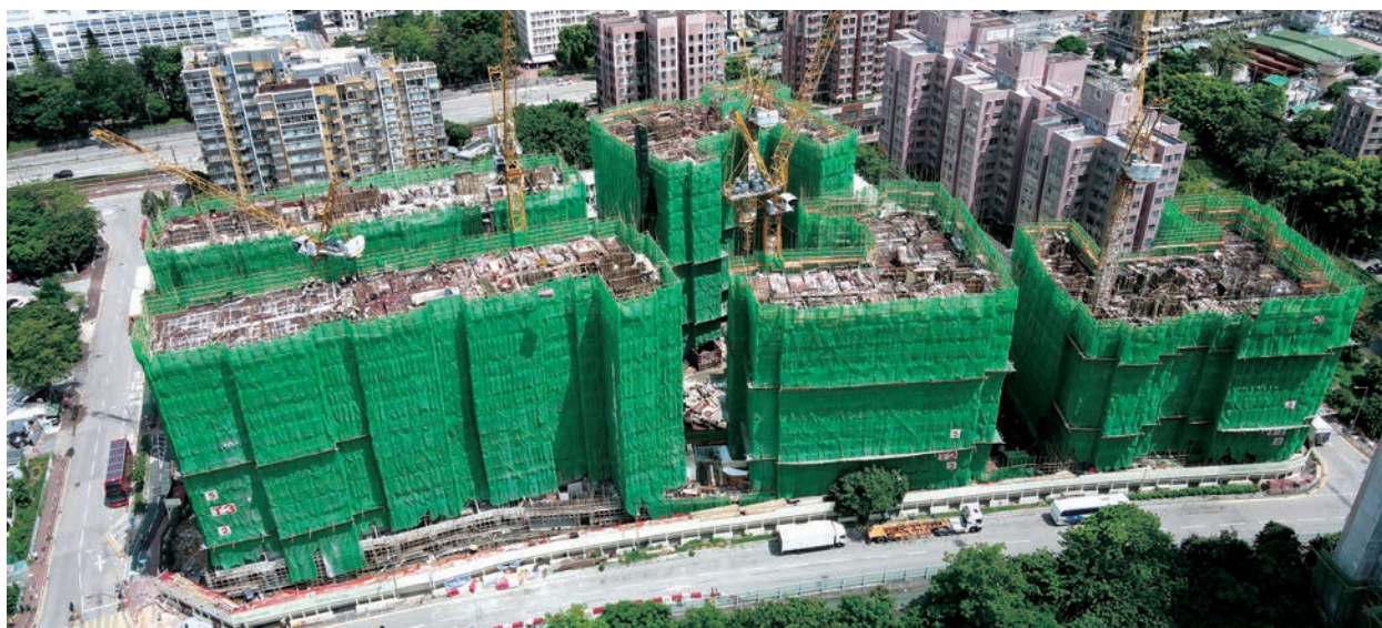
Residential development “High Park” in Hung Shui Kiu, Yuen Long
