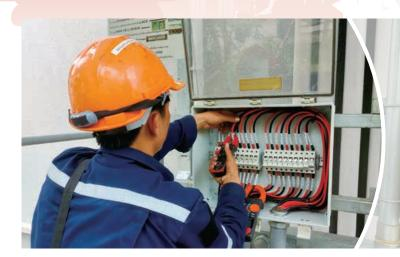
An RPCL worker performs preventive maintenance fuse checks for a solar rooftop project at an administration building.
