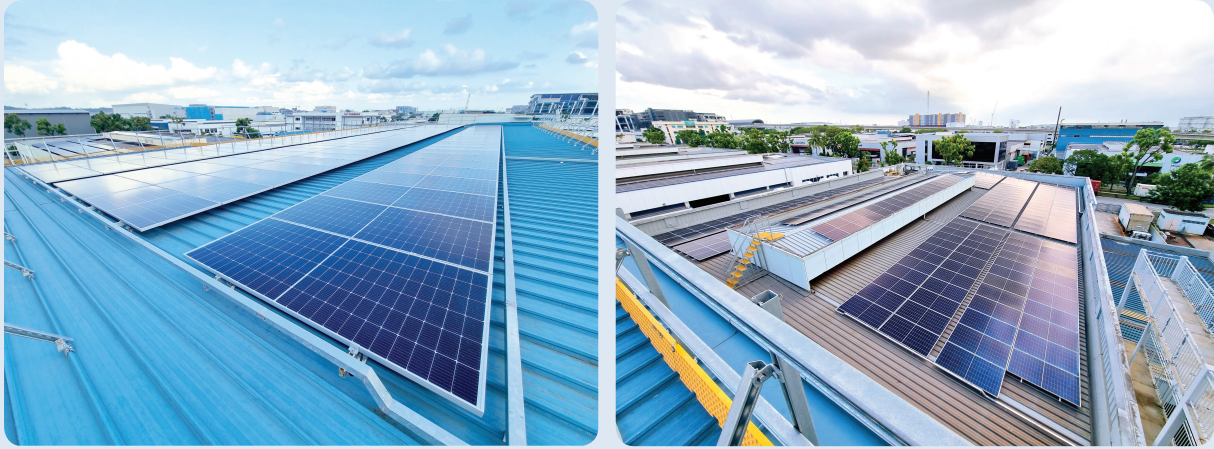
The rooftop solar systems
