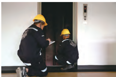
電梯服務 Elevator Services
