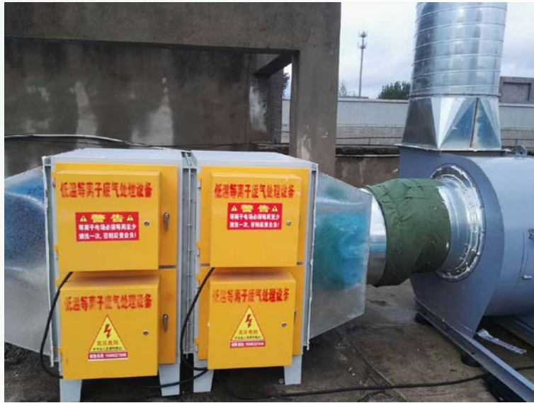
Low temperature plasma waste gas treatment equipment 低溫等離子廢氣處理設備
