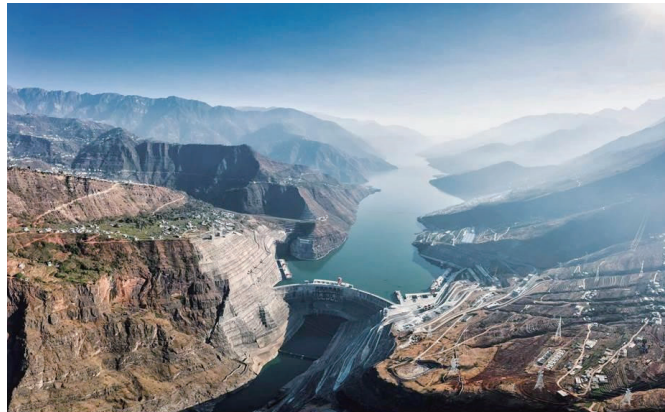
Ping An provides strong financial support for Baihetan Hydropower Station.
