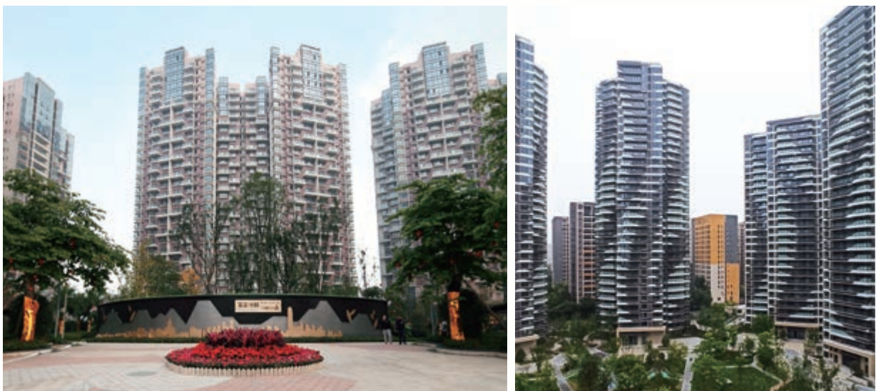
Casa Regalia (Phase 1 and Phase 2), Regal Cosmopolitan City - completed
