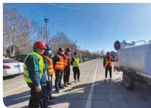
Using water mist gun trucks to reduce dust
