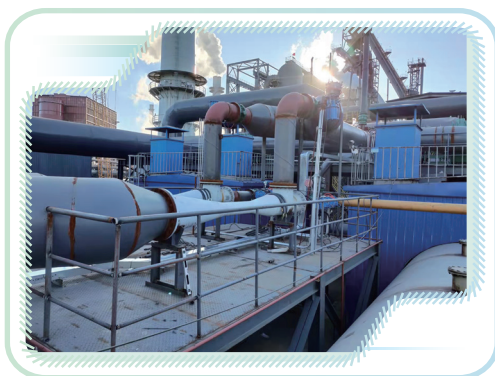
Equipment for blast furnace taking-off blast gas recycling 高爐休風放散回收設備
