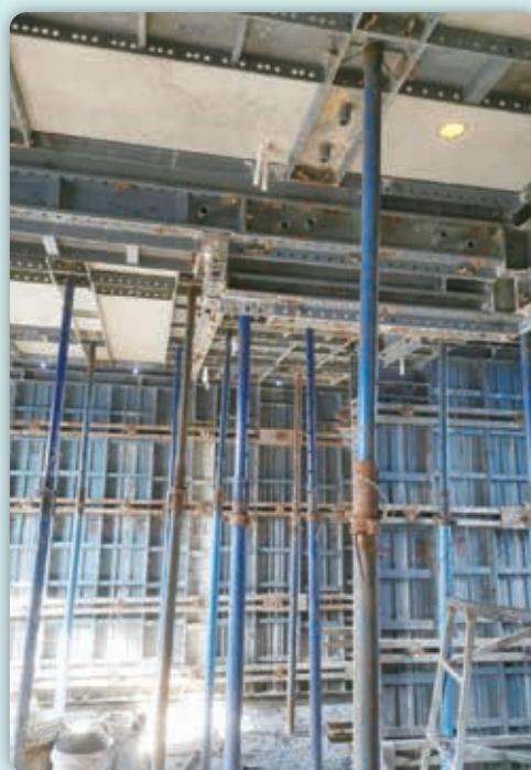
Aluminium formwork
