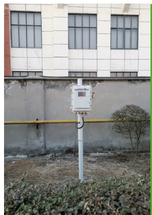
The plant is equipped with air VOCs monitoring equipment
