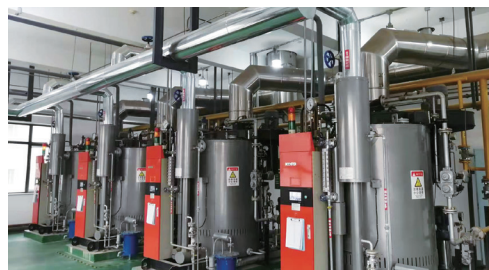
Low-nitrogen burners used for the gas-fired boilers in Beijing plant
