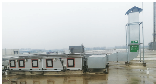
Tail gas treatment unit at laboratories in Beijing plant
