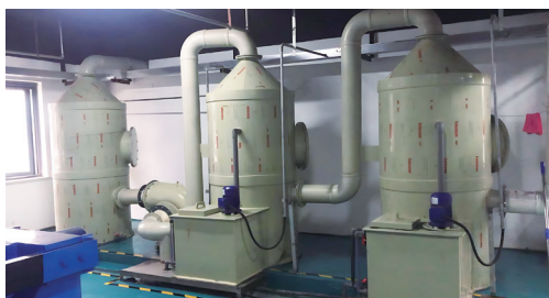
Harmless treatment of waste gas used for the sewage treatment system in Beijing plant
