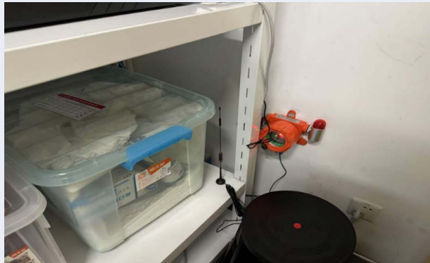
Pictured: Flammable gas alarm
