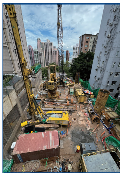
• 1 Kotewall Road project
